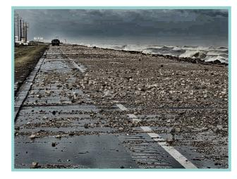
Highway 87 is a hurricane evacuation lifeline for the residents of the Bolivar Peninsula. This highway continually washes out and is in dire need of being raised to avoid flooding during weather events and high tides. While TXDOT has made improvements, additional work is needed to ensure resilency.
